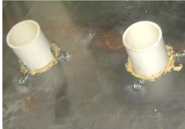
Figure 52: PVC Grout Holes
