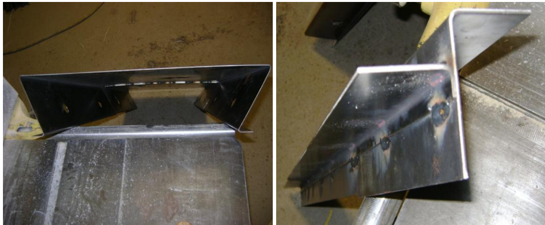
Figure 31: Fabricated Pieces before Installation
