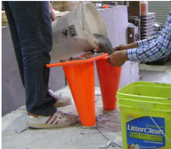
Figure 61: Pouring of Channel
